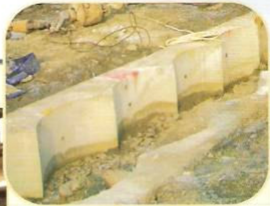
切削排樁導溝施作
